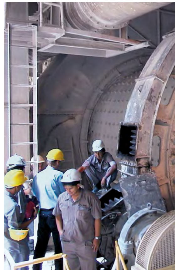
Inspection of a Ball Mill in a cement plant
