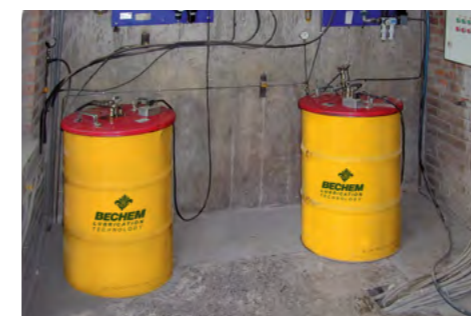
Drums of Berulit GA 2500 connected to spray systems
